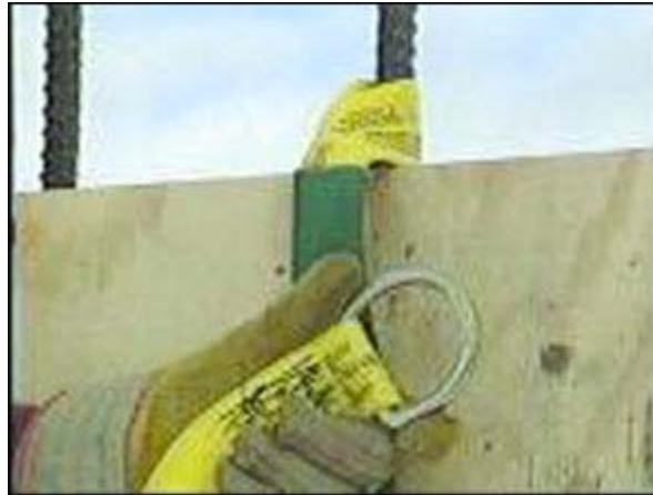
Figure 15 - A worker placing a strap on anchor over rebar.
