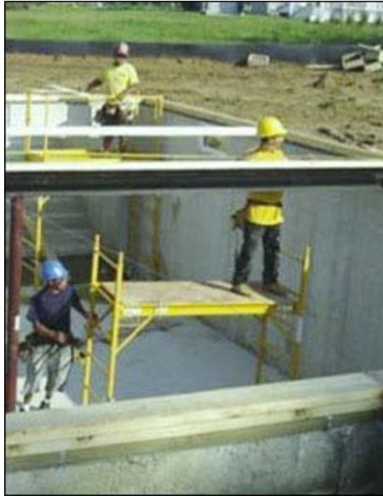
Figure 18 - Workers installing a steel beam from a mobile scaffold.
