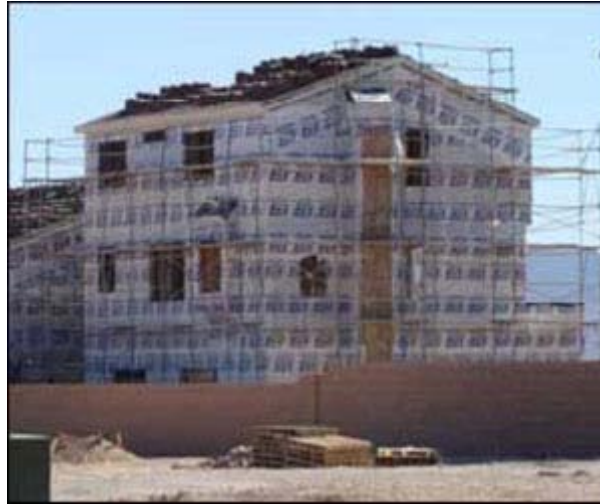
Figure 28 - Welded end frame scaffold.
