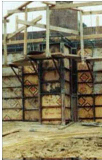
Figure 16 - A bracket-form scaffold attached to formwork.
