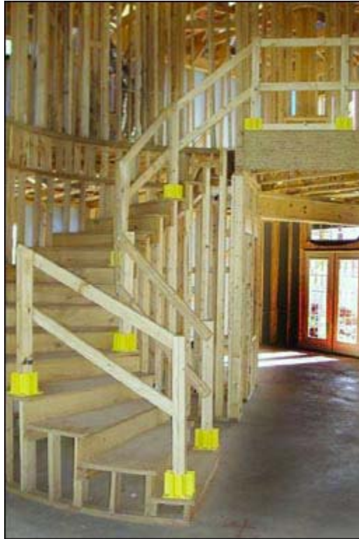
Figure 33 - Wooden guardrail system for a stairway.
