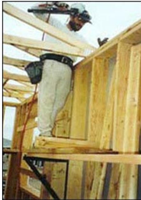
Figure 1 - A worker installing roof trusses from an interior bracket scaffold.
