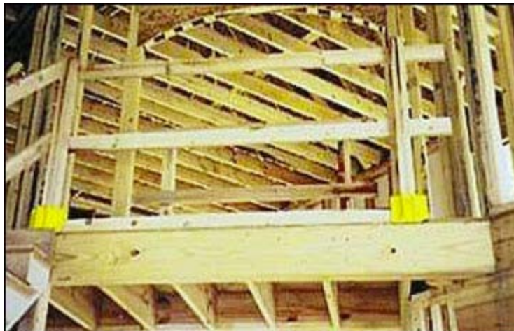
Figure 34 - A landing protected by a wooden guardrail system with a toeboard.
