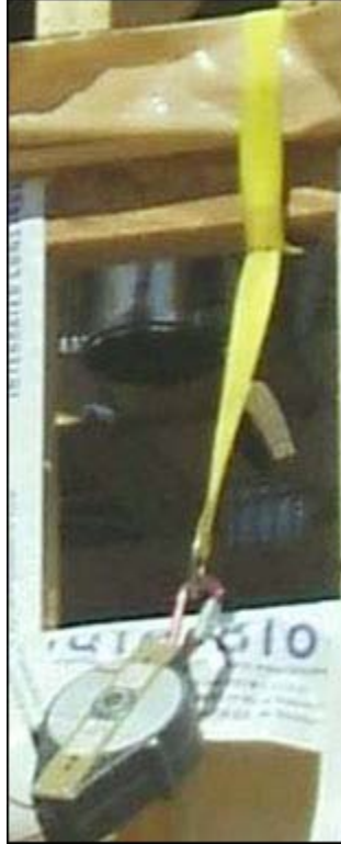
Figure 24 - A reusable strap anchoring a retractable lifeline.
