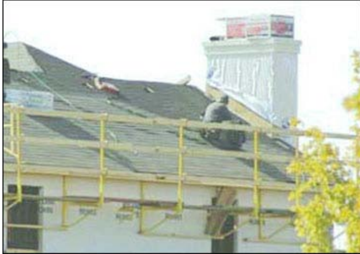
Figure 10 - An exterior bracket scaffold with guardrails being used to protect workers while weatherproofing.
