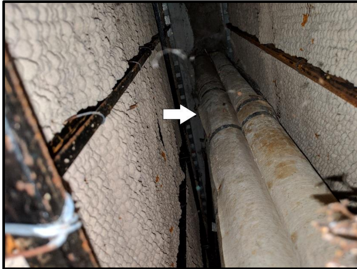
ACM pipe insulation
