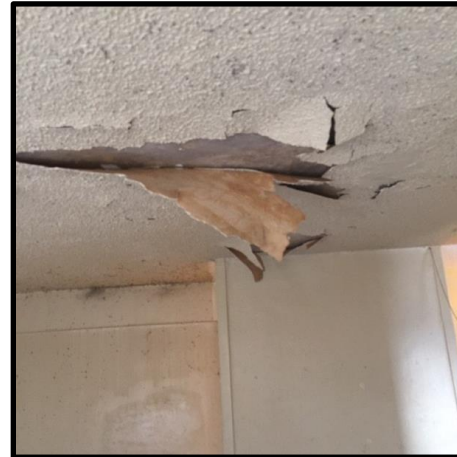
Close Up: Living Room Ceiling
