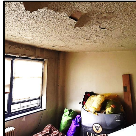
Full View: Living Room Ceiling
