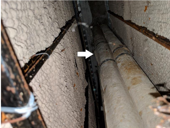
ACM Pipe insulation
