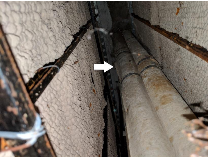
ACM- Pipe insulation (T.S.I)
