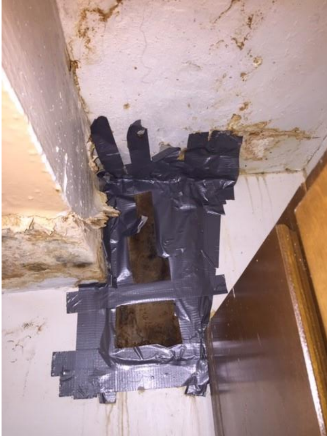
Close Up: Kitchen
