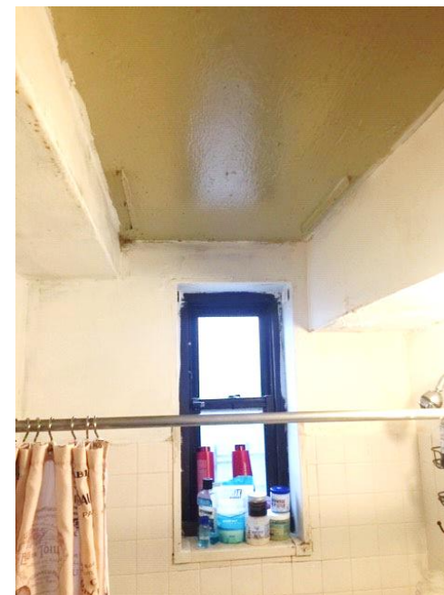
Full View: Bathroom Wall
