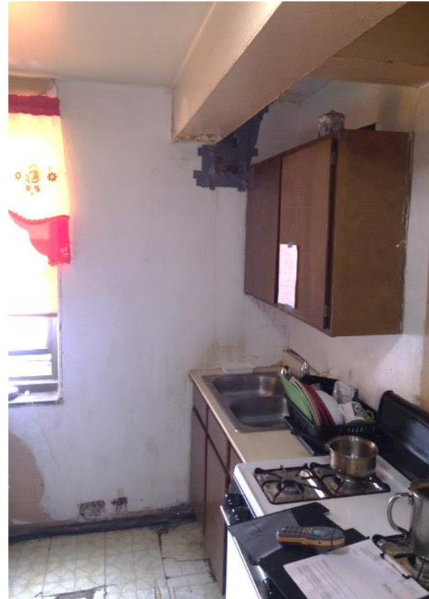
Full View: Kitchen
