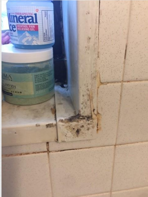
Close Up: Bathroom Window Frame
