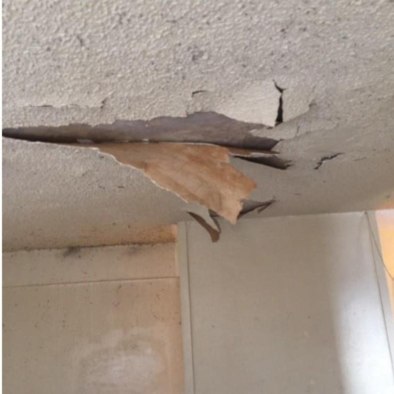
Close Up: Living Room Ceiling
