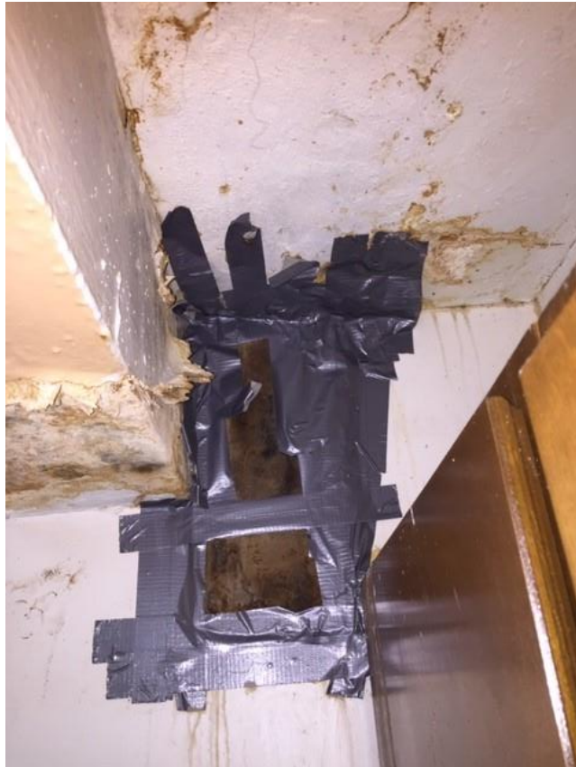
Close Up: Kitchen
