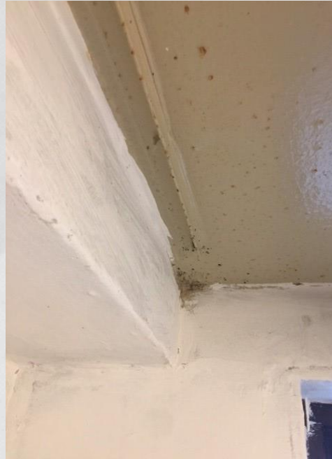
Close Up: Bathroom Ceiling
