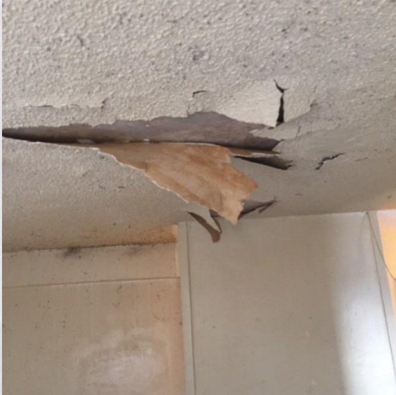
Close Up: Living Room Ceiling
