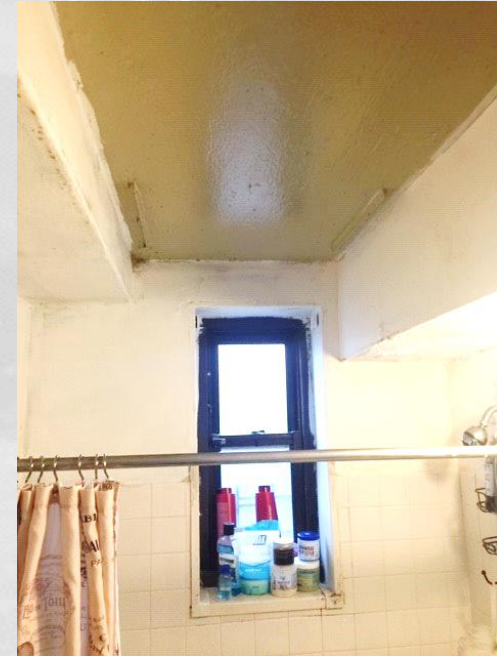
Full View: Bathroom Wall
