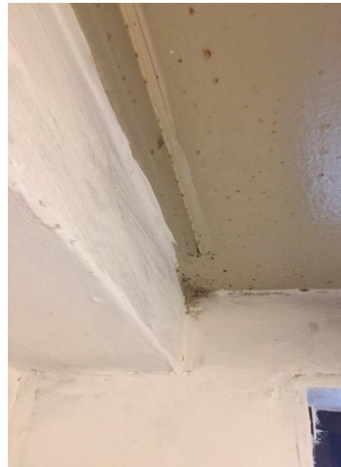
Close Up: Bathroom Ceiling
