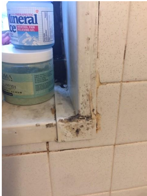
Close Up: Bathroom Window Frame
